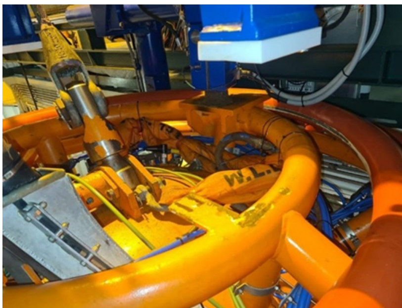
Main Bell Wire with spelter socket, Connection Swivel and Bell Flanges, Overview
