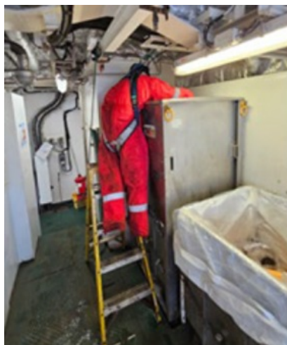
Position of person while reaching into compactor (re-enactment)
