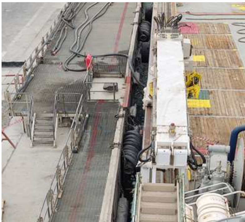
View of the spillage area in the morning
